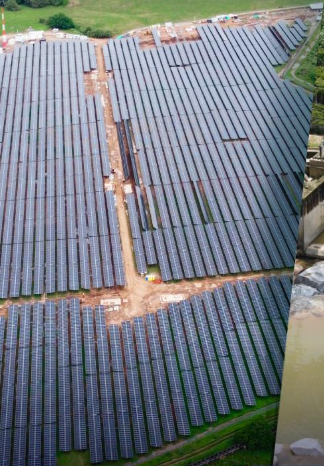
Brisas solar park (26 MW)
